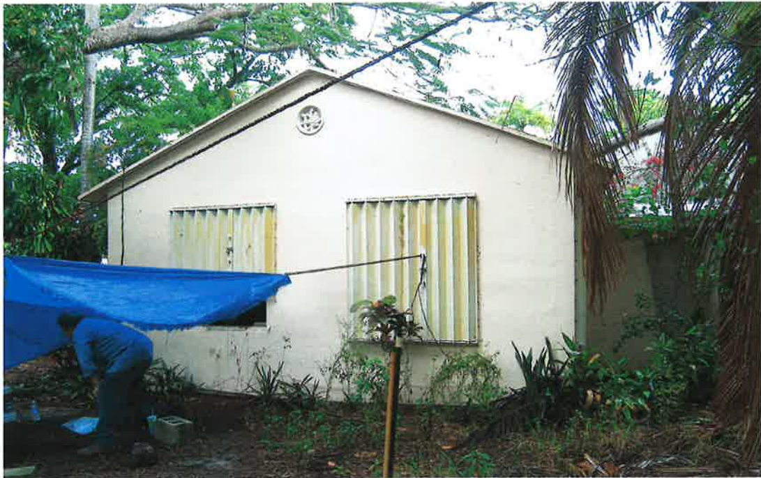
8BD04547: above, cottage front, looking southeast; below, cottage looking east.
